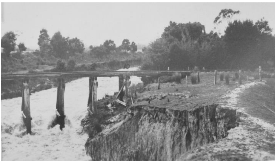
Lang Lang Straight Cut bridge closed by this erosion in 1942
