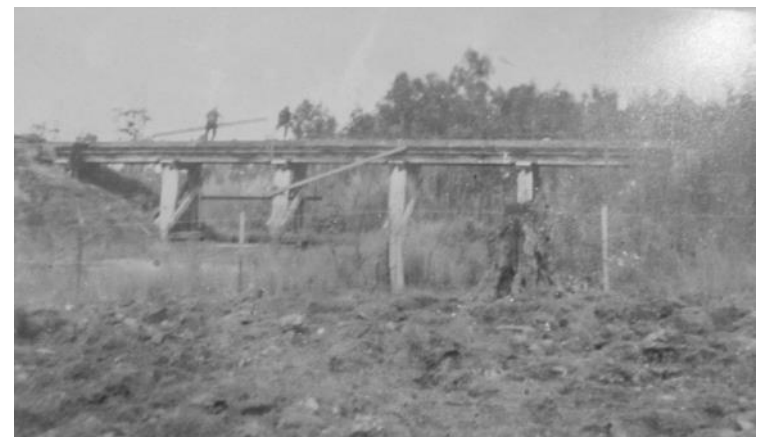
Crompton's Creek bridge between Heathhill and Athlone Image; On display at the Back-to Bayles celebration in June 2022
