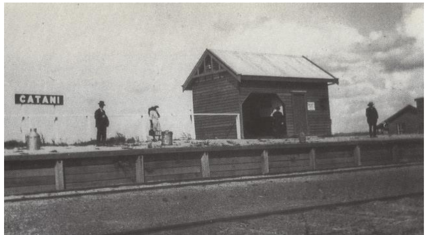
Catani Railway Station
