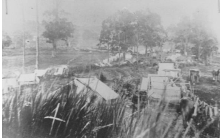
Construction camp near Strzelecki in 1921-22 Image; On display at the Back-to Bayles celebration in June 2022
